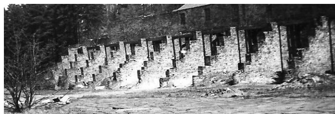
Bouse teams (also known as Bingsteads) used to store the ore (Photographed at Allenheads courtesy of Mr and Mrs Handcock)
