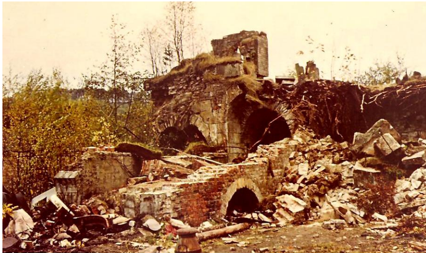
Arches supporting flues at Allen Mill, Photograph taken 1973 (Courtesy of Mr and Mrs Handcock)
